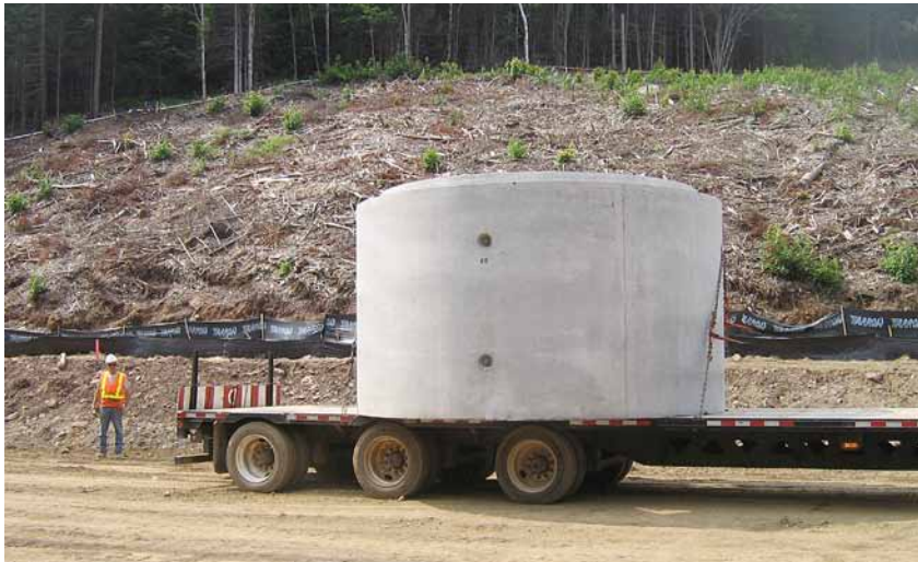
Because of its weight, each section of culvert required its own flatbed trailer.
