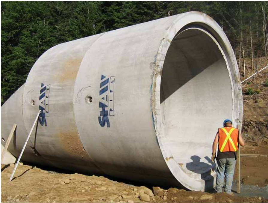
At left is the endpiece of one of the pipes where Manzer Brook will exit into the open. The end is shaped much like the spout of a pitcher. Imagine it buried in earth that is sloped at the exit to match the angle of the "spout."
