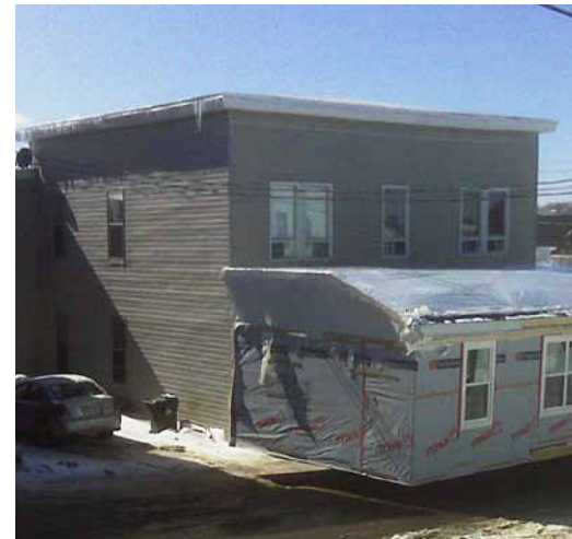
A 70-foot module works its way through icy Saint John streets. Construction started in December 2008 and ended in July 2009.
