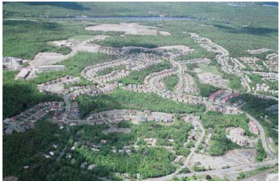
First, lines on a plan, then rough dirt tracks on the hillside. Now large parts of The Ravines of Bedford South are landscaped streets of finished homes.
