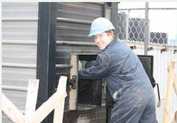
Colin Mills stokes the furnace with waste wood from discarded pallets.
